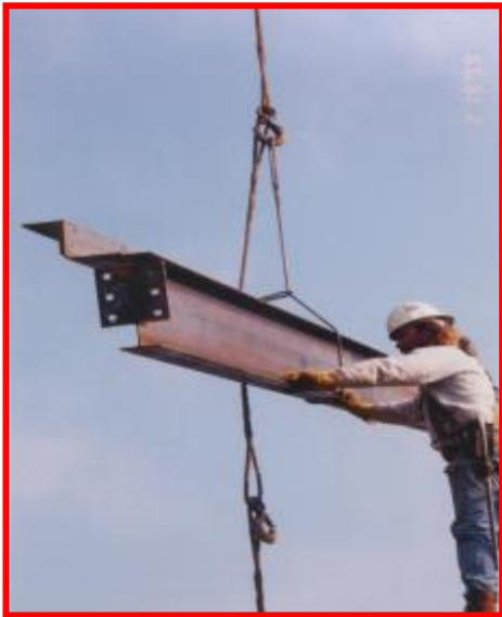
The connector in the illustration on the left is safely lowering the load and ensuring the hooks do not contact himself or the beams. Training is the keystone of our organization and the Ironworkers National Training Fund has developed a nationally recognized "Qualified Rigger Program" and is working on the development of the "Rigger Certification Program".
